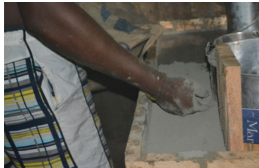
66 Agregando cemento gris
